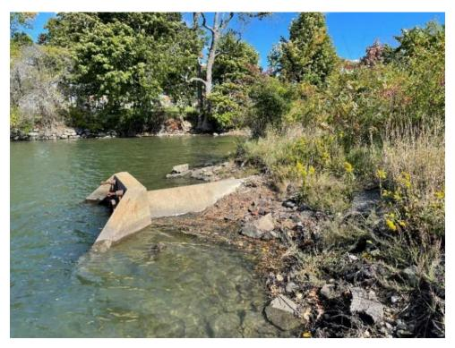
Photo 3 – Existing outfall headwall, exposed 48" RCP pipe, and tidal embankment looking east at approximate high tide. Taken 9/28/22
