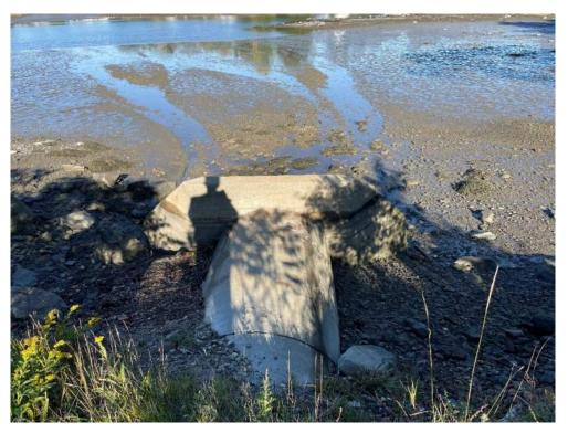
Photo 5 – Existing outfall headwall and exposed 48" RCP pipe looking northwest at approximate low tide. Taken 9/29/22
