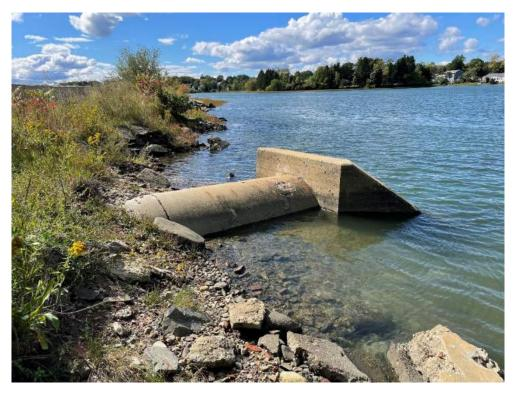
Photo 1 – Existing outfall headwall, exposed 48" RCP pipe, and tidal embankment looking west at approximate high tide. Taken 9/28/22
