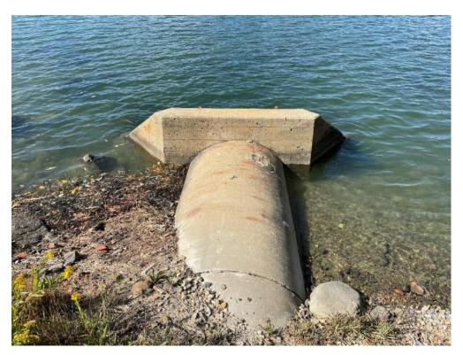
Photo 2 – Existing outfall headwall and exposed 48" RCP pipe looking northwest at approximate high tide. Taken 9/28/22
