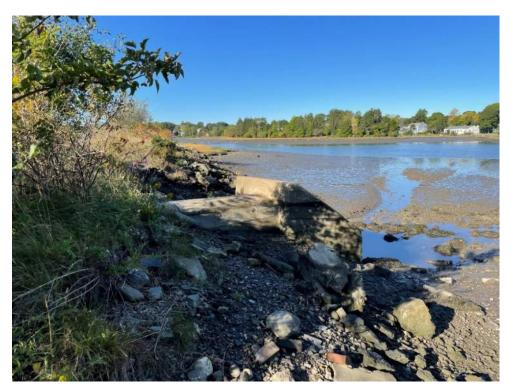
Photo 4 – Existing outfall headwall, exposed 48" RCP pipe, and tidal embankment looking west at approximate low tide. Taken 9/29/22
