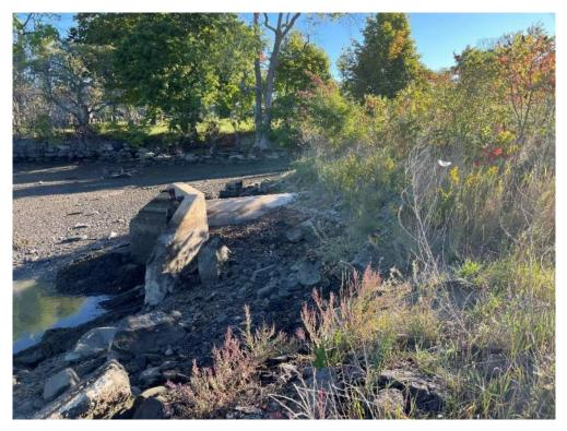
Photo 6 – Existing outfall headwall, exposed 48" RCP pipe, and tidal embankment looking east at approximate low tide. Taken 9/29/22
