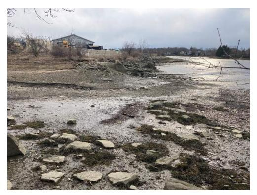
Photo 8 – Mitigation area, looking southeast at approximate low tide. Note existing large rocks to be stockpiled for use on stabilized slope and ice breakers. Taken 3/20/24
